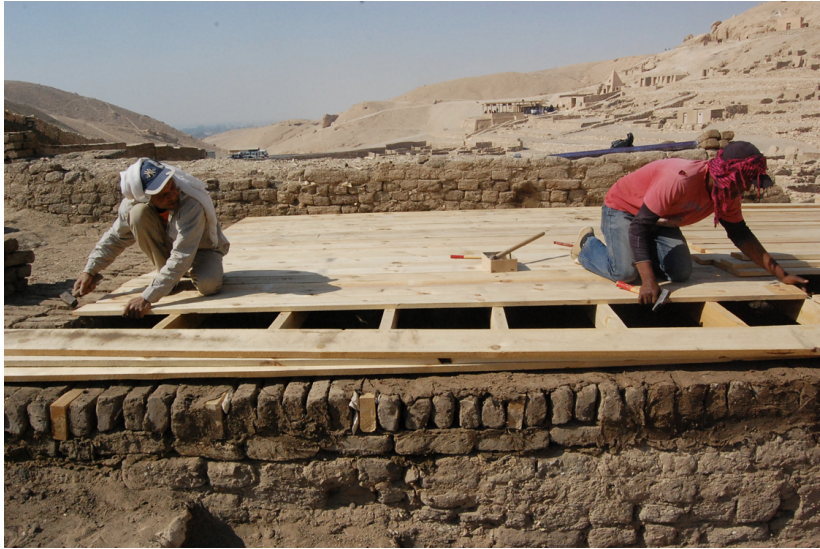
Restoration of the ceiling of the chapel located against the north wall of the village (2012 campaign)..
