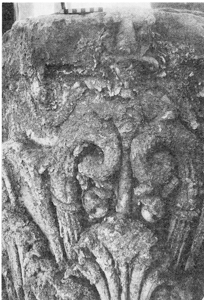
5. The salt efflorescence on the Hellenistic capitals.
