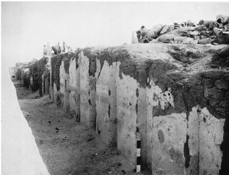
FIG. 12. Mastaba Saqqara 3505 (1st Dynasty), West façade of the superstructure from the south, Emery et al. 1958, pl. 15a.
