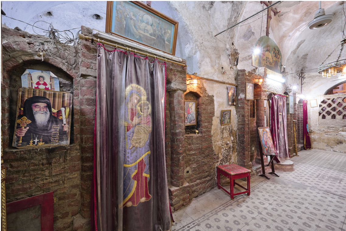
FIG. 12. The brick altar screens constructed in the church of Dayr Abū Ḥinnis in the 1940s.
