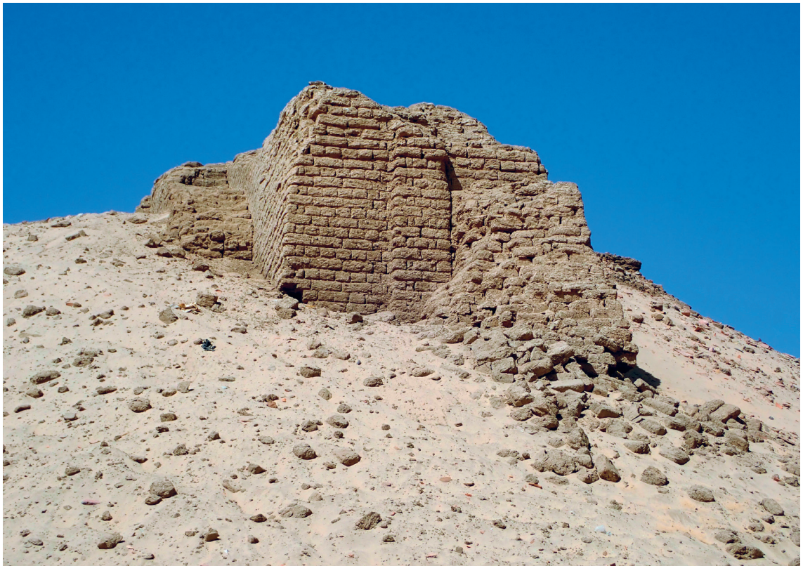
FIG. 27. South end of M438 showing blocking wall M452, staircase M439, looking north.
