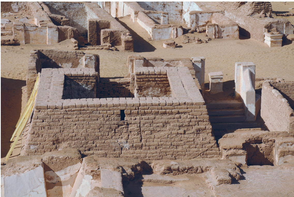
FIG. 22. The exterior opening of the air hole of the burial chamber.
