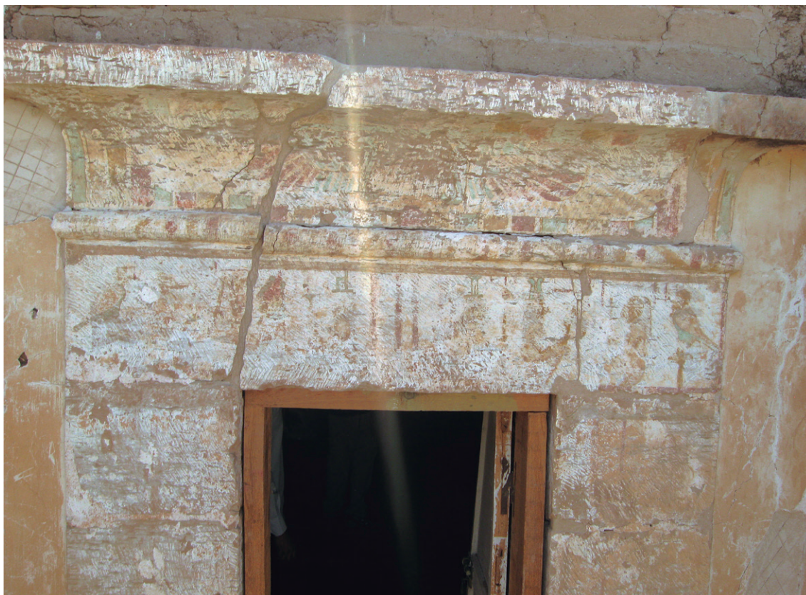
FIG. 19: Bir el-Shaghala Tomb 1, ground floor: painted entrance lintel.
