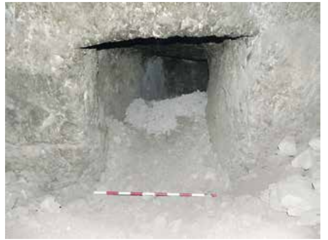
Pl. 2d. Tunnel filled with debris.
