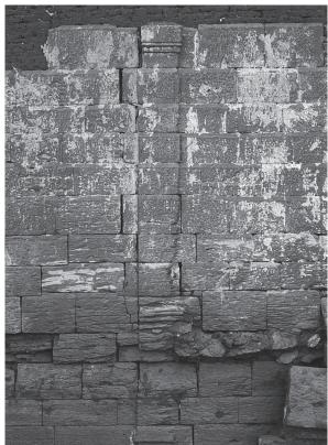
Photo 9. Tomb 4, east side. A pilaster. Traces of plaster.
