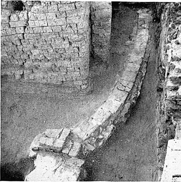
44. Corridor est, canalisation.
