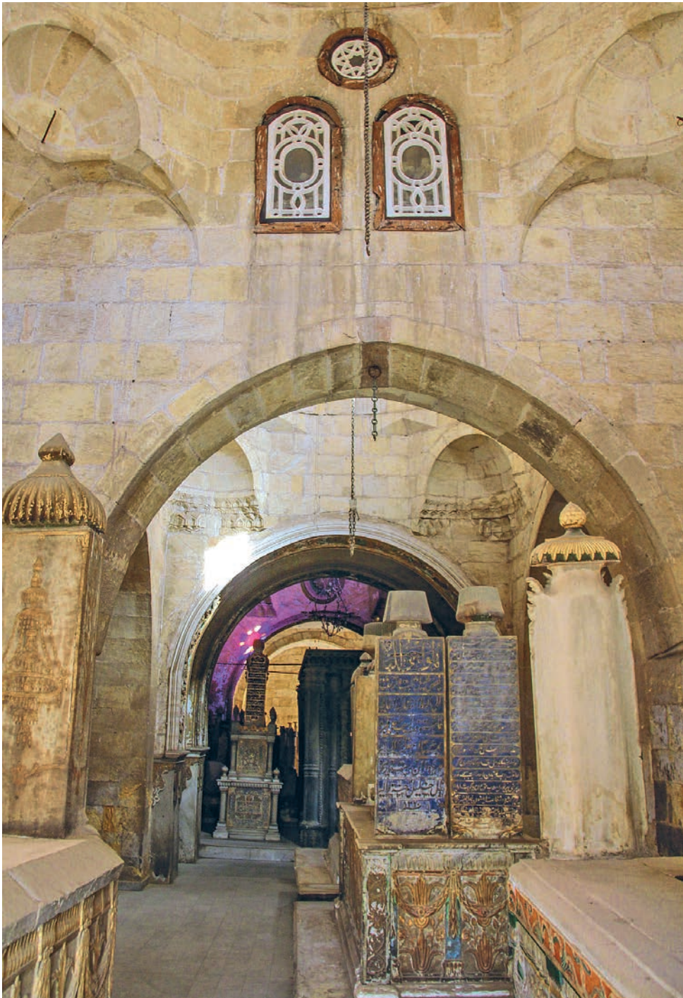
Fig. 6. Interior view from Amīna Hānim's dome chamber looking towards Ismā'īl Pāshā's chamber, followed by Ṭūsūn Pāshā's chamber; the windows between the trilobed arches are purely decorative and filled with rubble masonry (Photo: Mai Kolkailah).
