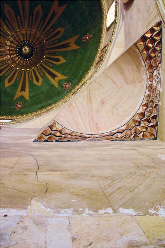
Fig. 30. Imitation marble dado on the northeastern wall in Ibrāhīm Pāshā's dome chamber (Photo: Mai Kolkailah).
