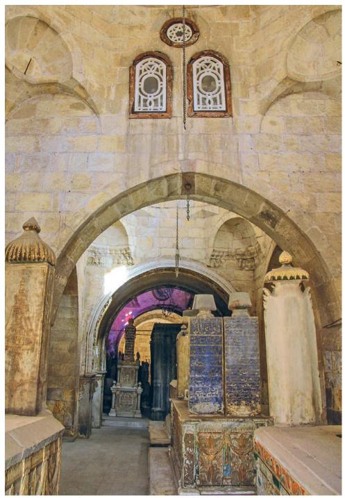
Fig. 6. Interior view from Amīna Hānim's dome chamber looking towards Ismā'īl Pāshā's chamber, followed by Ṭūsūn Pāshā's chamber; the windows between the trilobed arches are purely decorative and filled with rubble masonry (Photo: Mai Kolkailah).
