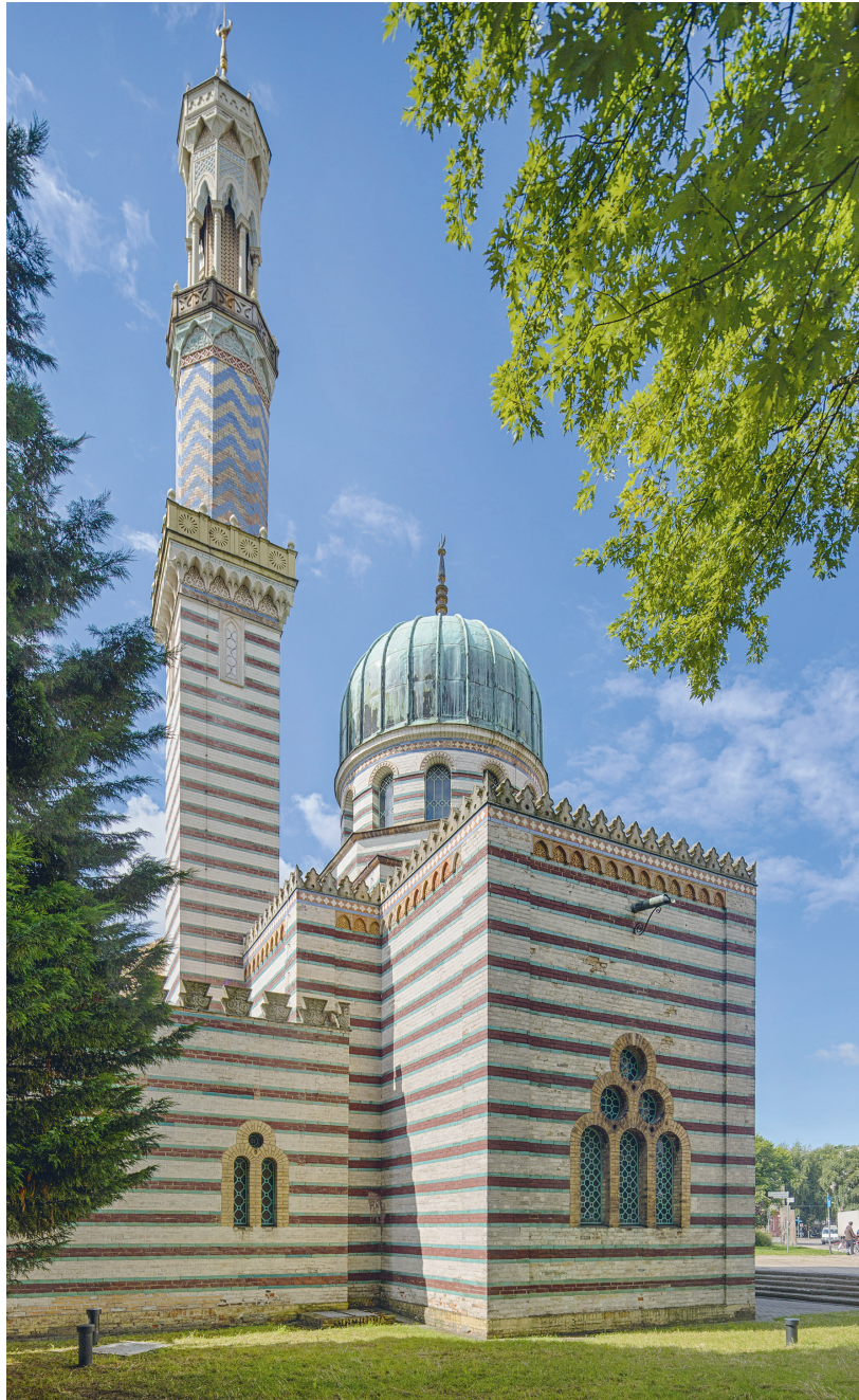
Fig. 1. Potsdam, pump station of Sanssouci palace, by Ludwig Persius, 1841–1843 (photo: B. O’Kane, 2013).
