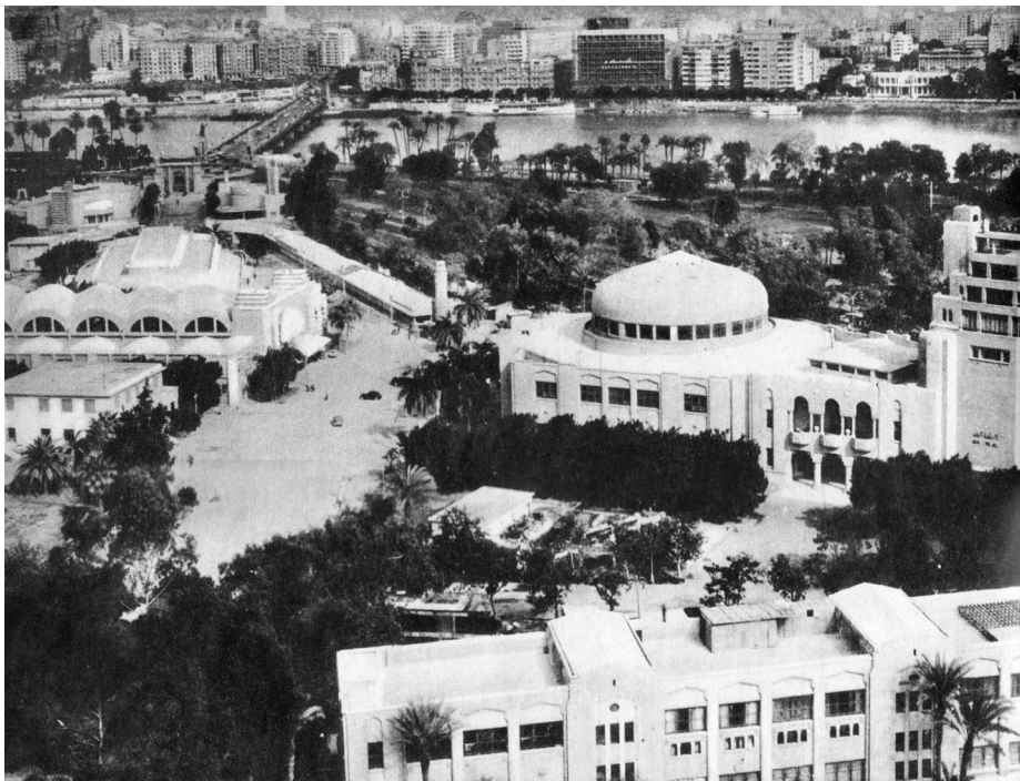
Fig. 5 Aerial view of the exhibition grounds circa 1958. In the center left are the Agriculture Palace (front) and the Industry Palace (back), The Grand Palais is to the right and the Petit Palais is partially shown in the bottom of the photograph. Published in Binā' al-Waṭan , February 1960.
