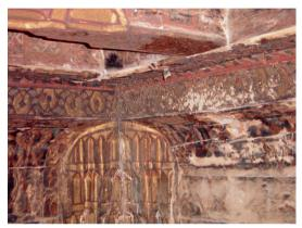
Fig. 1. General view (up left), Façade (up right) and ceiling (down) showing the effect of air pollution and dust on the wall paintings of the Sabil Alkazlar.
