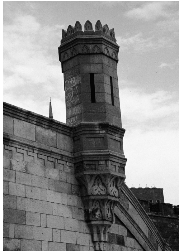
Fig. 4. Bab al-Azab renovated by Khedive Ismail circa 1870. Miniature towers in Revival Style.
