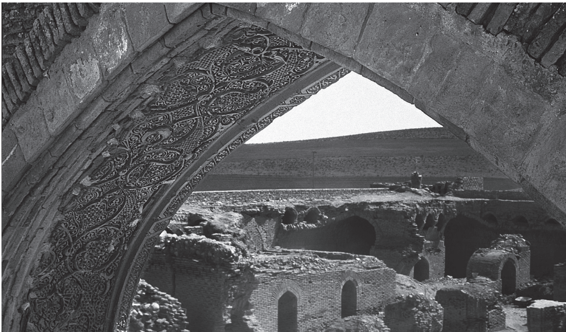
9. Ribāt-i Šaraf, arch of main iwān (photograph by the author).
