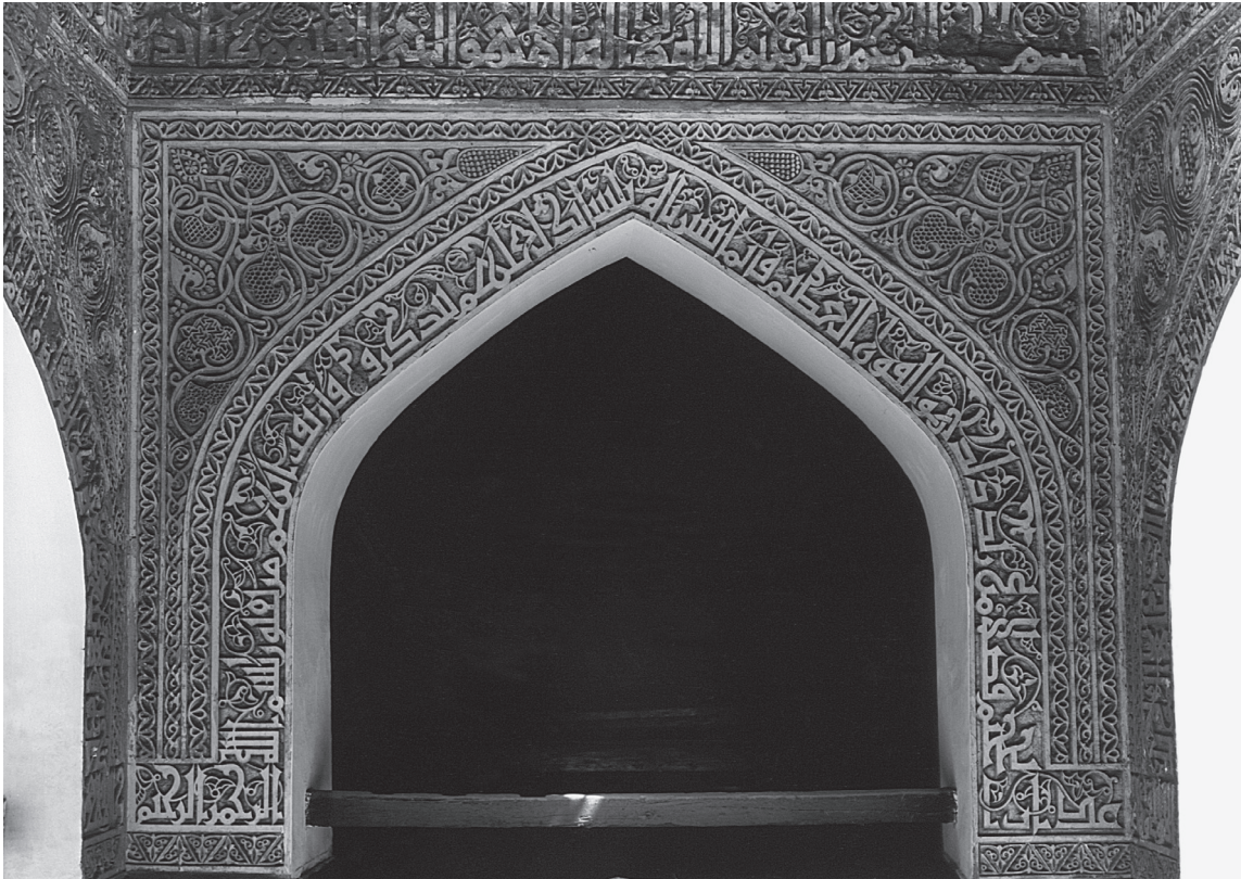
2. Cairo, al-Azhar Mosque, arch under transept dome (Ashmolean Museum, Oxford, Creswell Archive no. C.3046).
