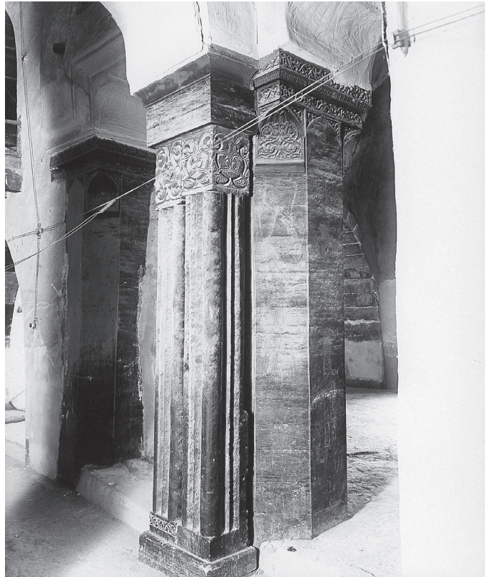
6. Mosul, Mosque Al-Nūrī: Type 2 column placed against type 1 column, condition c. 1930. (Courtesy of the General Institute for Antiquities, Baghdad).
