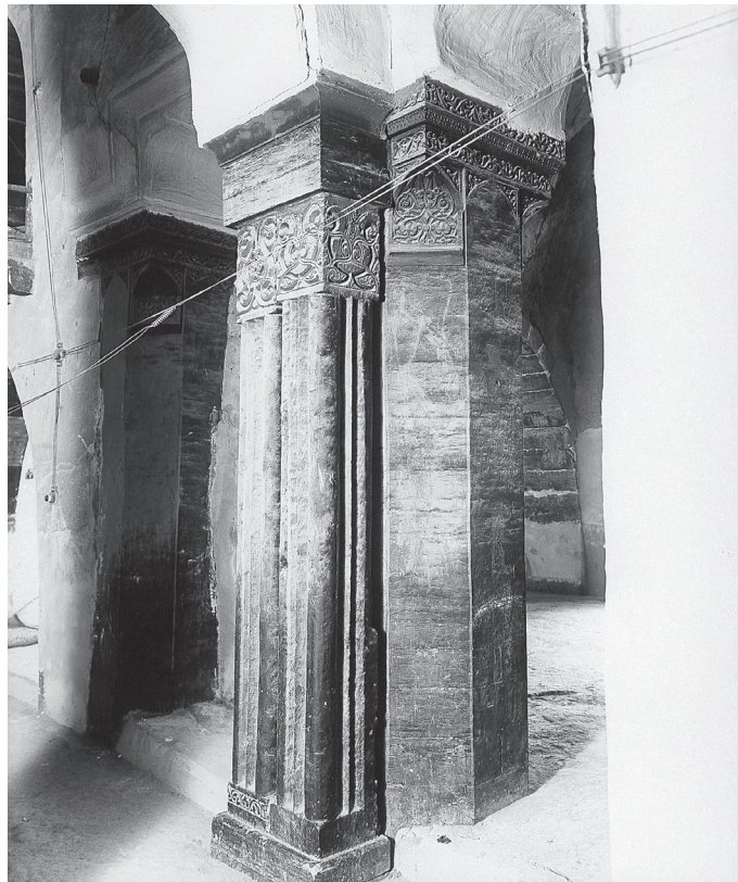
6. Mosul, Mosque Al-Nūrī: Type 2 column placed against type 1 column, condition c. 1930. (Courtesy of the General Institute for Antiquities, Baghdad).
