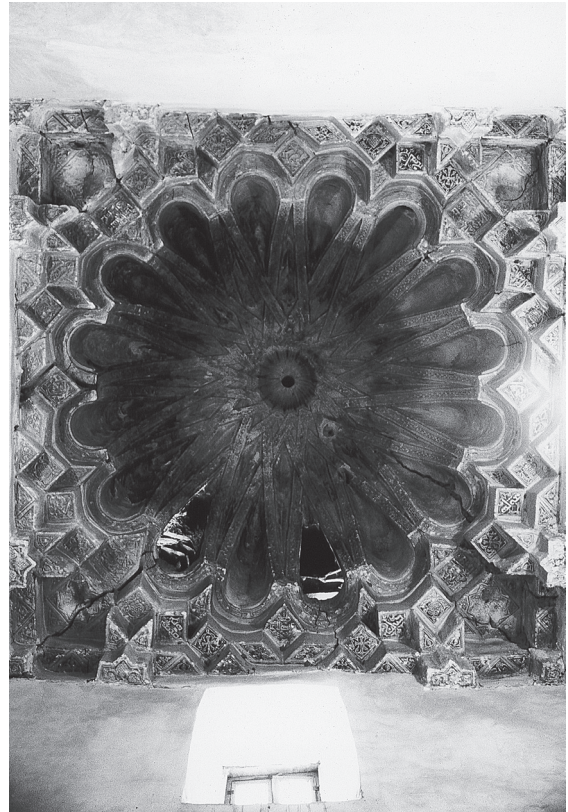
13. Mār Behnām near Mosul: Ribbed vault over the Chapel of the Virgin, first half of the thirteenth century.
