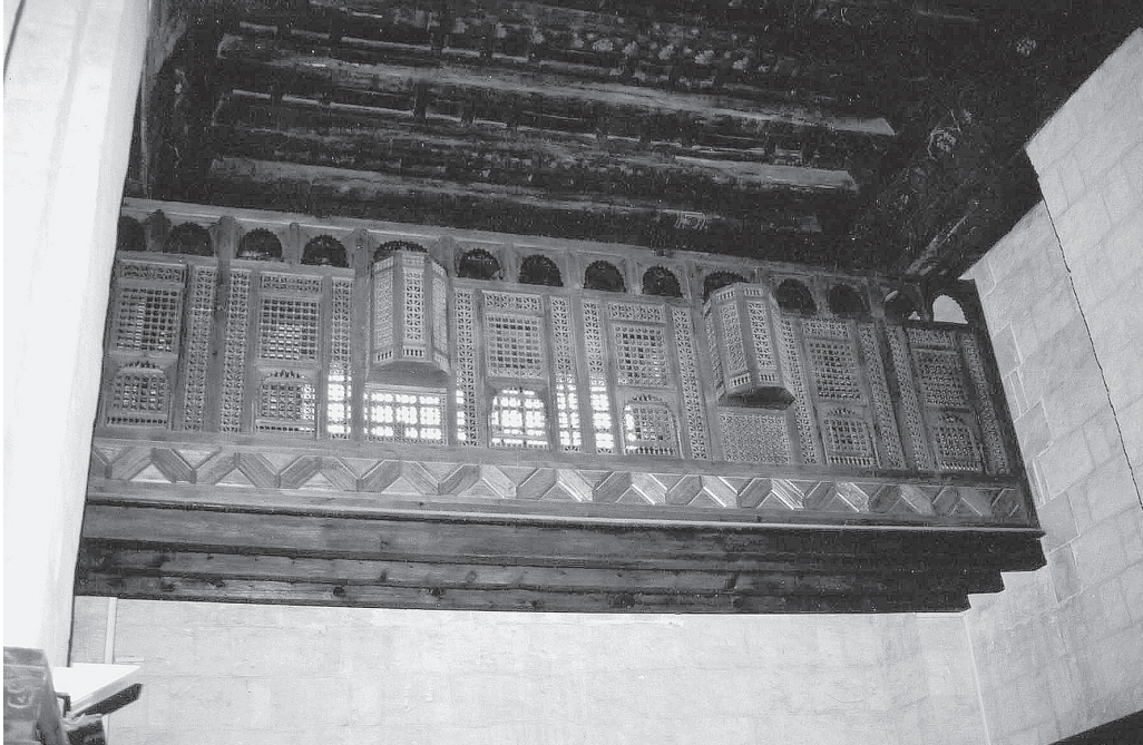
12. Bayt Mustafa Ja'far, Bridge crossing the ground floor qa'a at mezzanine level.
