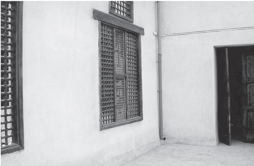
13. Bayt Mustafa Ja'far, Lobby 16 on the first floor.
