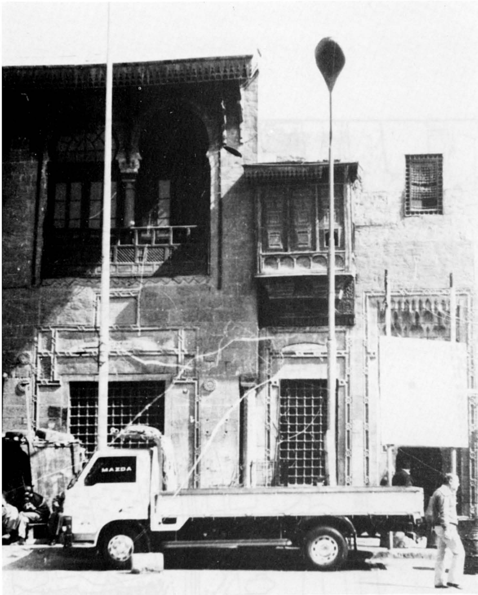
Fig. 2. Sabil-kuttab of al-Hajj Bashir Agha. Monument No. 309. 1131 A.H. / 1718 A.D.
