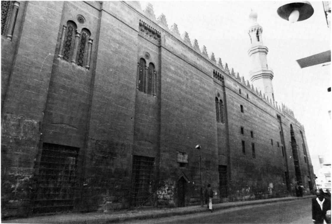
a. — Façade of the Hānqāh of Šaiḥū.
