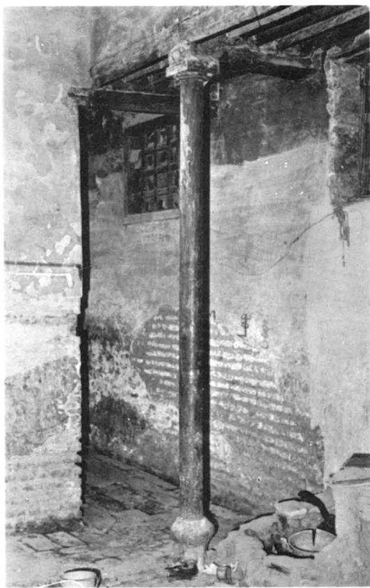
A. — First unit south staircase : wooden column near passage leading to the latrine.
