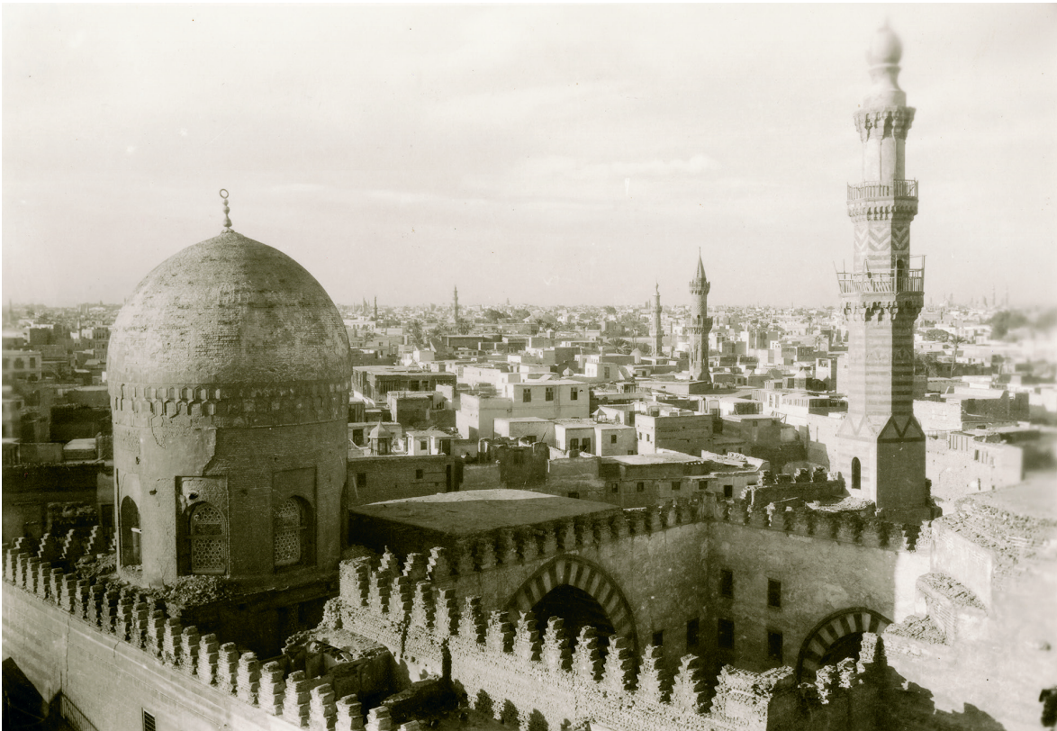
Fig. 8. Unknown photographer, [Mosque and minaret of the mosque of Şarġatmiş], post 1894 and before 1935. Silver print, Creswell Photographic Collection, The American University in Cairo. Album 22. Courtesy of RBSCCL.
