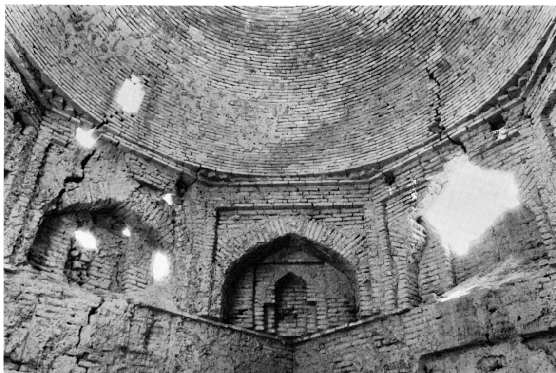
b. — Ribāṭ-i Sāḥib Zāda, Hānqāh of Ġalāl al-Dīn Aḥmad : interior, zone of transition.
