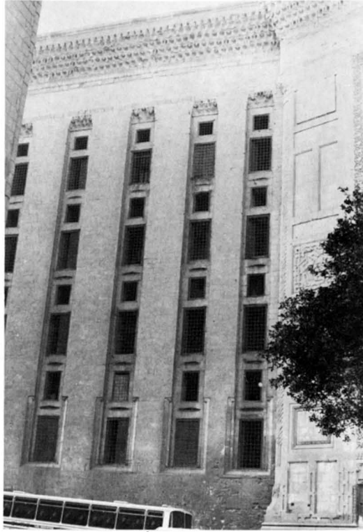
a. — Façade of the Madrasa of Sultan Ḥasan with living units overlooking the street.
