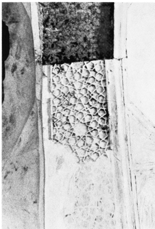
b — Ġalvār, Masġid-i Hauḍ-i Karbās, soffit of transverse arch.
