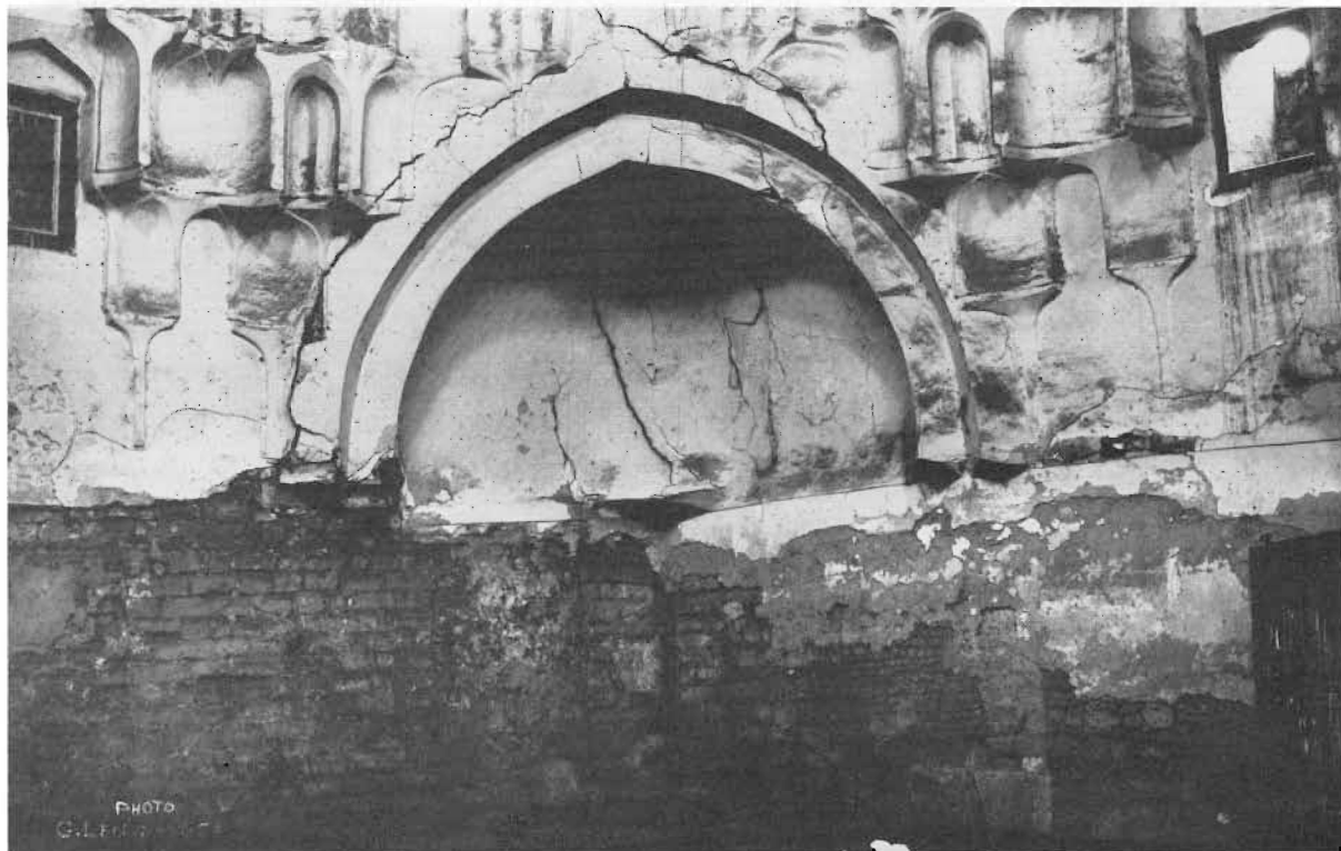
B. — Squinch of the large dome of Ġānibak at Qaṣr al-ʿAynī.
