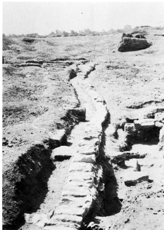
C. — Path of aqueduct through quadrants X-18/21/22 and XIV-1; looking SW.
