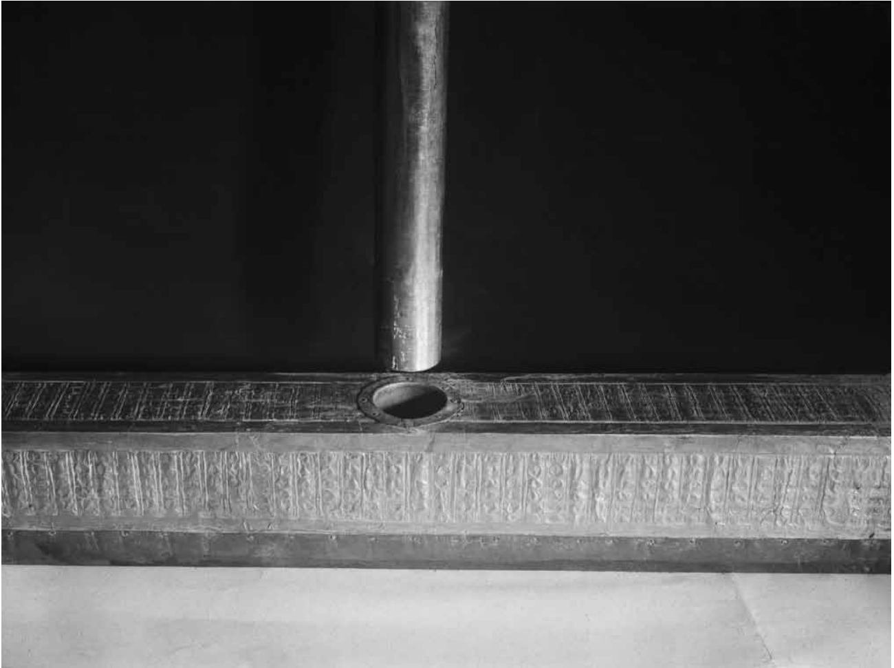
PL. 3. Base of pole and socket in floor beam. Photograph courtesy of the Museum of Fine Arts, Boston.
