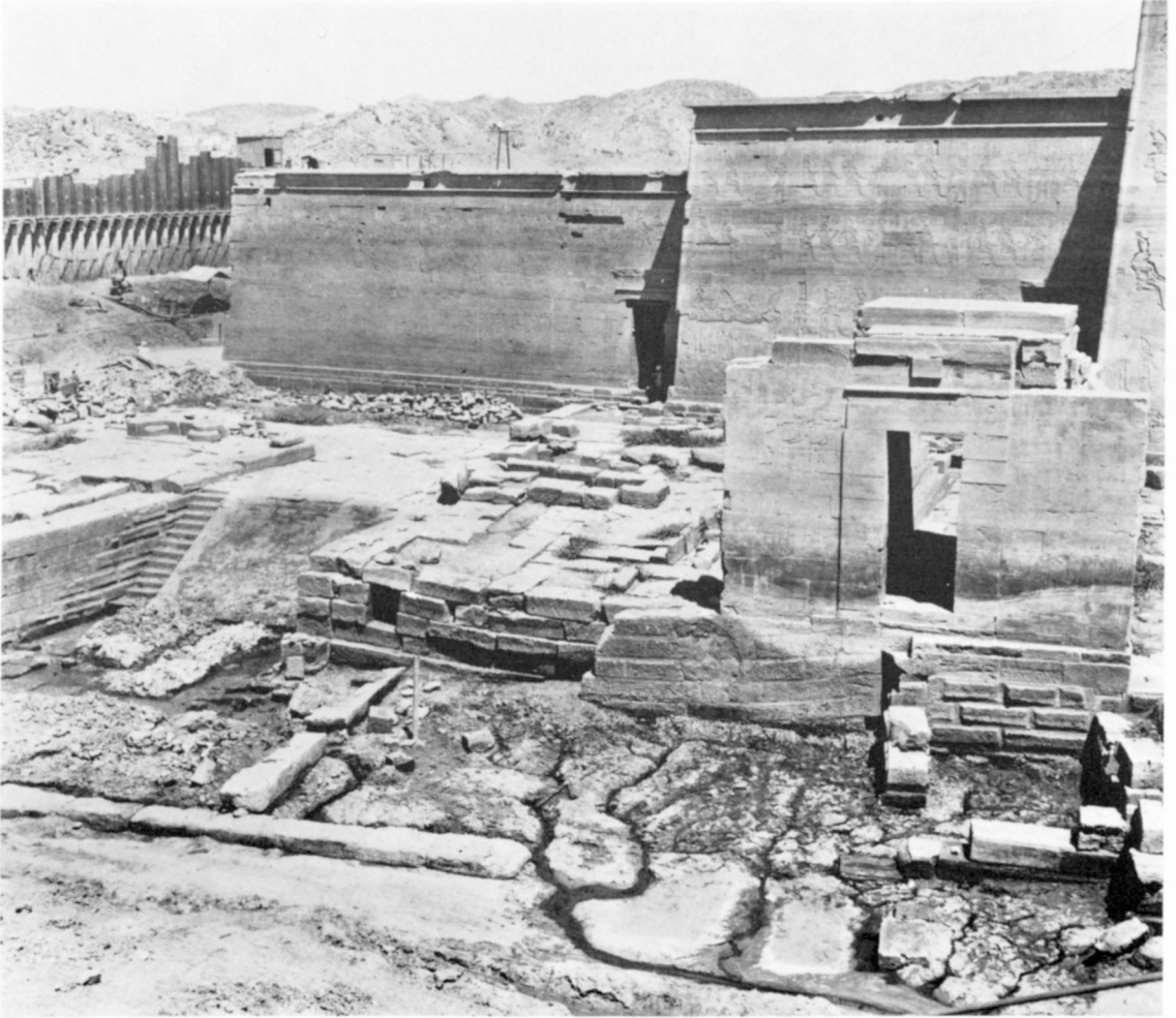
A part of the enclosure wall west of the Temple of Isis.
