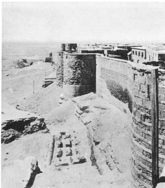
B. — Northern enclosure, east side, showing the Bâb al-Qarâfa and rock-cut ditch.
